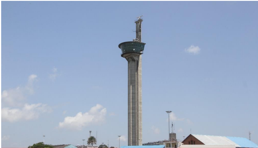
The Mombasa VTS Control Tower from where the activation signal was relayed
