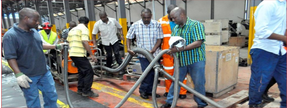
MR. SAHA HANDLES THE AIR BLOWER HOSES
